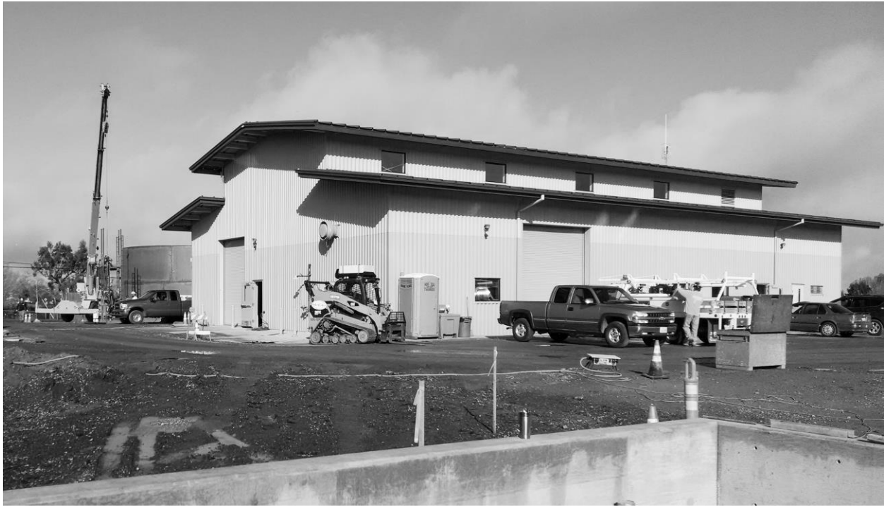
Lessalt Surface Water Treatment Plant Upgrade Construction
