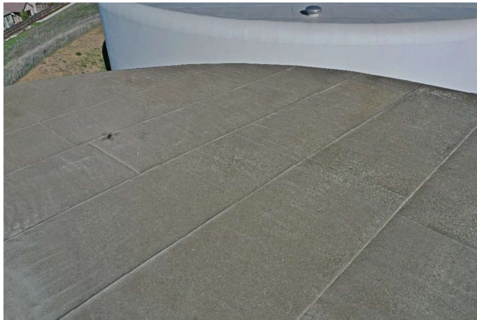
E-8 Same as Photos E-6 and E-7, except in a different location.
