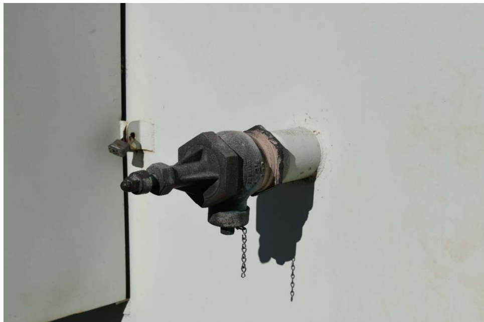
E-25 View of a small diameter penetration, illustrating generally good condition of the brass valve and adjacent paint system.
