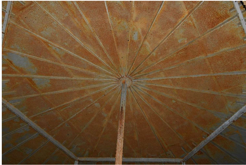
I-2 Same as Photo I-1, except a closer view of the inner bay.
