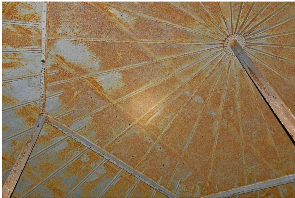
I-5 Same as Photo I-4, except a different portion of the inner bay.
