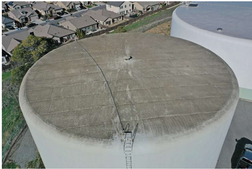
E-2 Same as Photo E-1, except a closer view of the roof.
