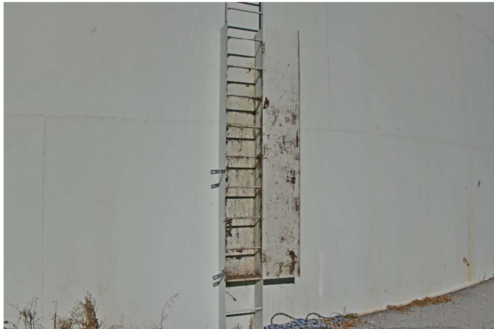
E-15 View of the bottom of the ladder, illustrating dirt and debris behind the ladder vandal guard and otherwise generally good condition of the paint system.
