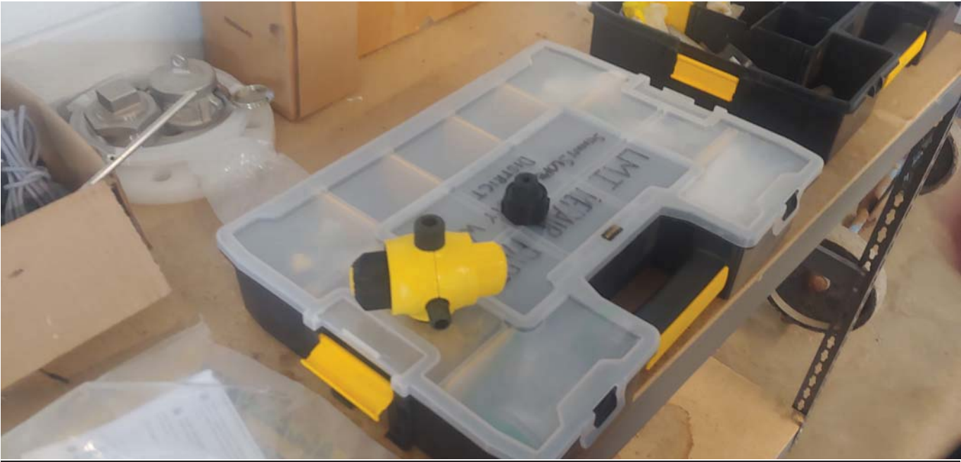
Routine Chemical Dosing Pump Maintenance, See description next page.
