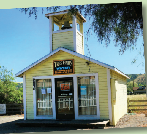
Tres Pinos Water District is one of three small local water providers that will be consolidated into the Sunnyslope system.
